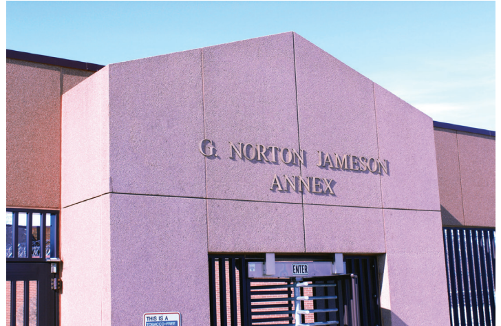
The G. Norton Jameson Annex at the South Dakota State Penitentiary in Sioux Falls. (John
