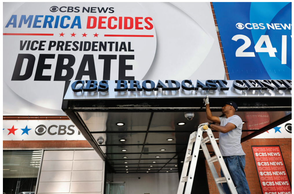
The entrance to the CBS Broadcast Center undergoes repairs on Sept. 30, 2024, the day before the vice presidential debate in New York City between Republican vice presidential candidate, Sen. J.D. Vance, R-Ohio, and the Democratic vice presidential candidate, Minnesota Gov. Tim Walz. (Chip Somodevilla/Getty Images)
