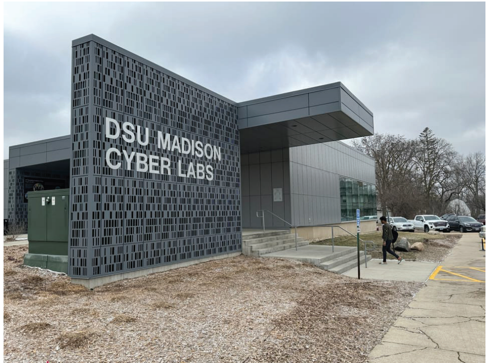
The $18 million, 40,000-square-foot MadLabs research facility, shown on the Dakota State University campus in Madison, S.D., on March 22, 2024, is a hub for cyber research. (Photo; Bart
