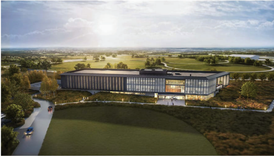
A rendering of DSU's Applied Research Lab (ARL) under construction in Sioux Falls, S.D. (Source: Dakota State University)
