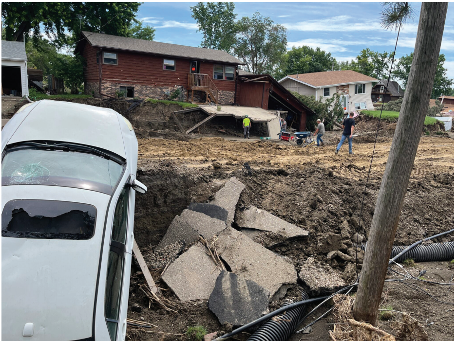
Damages remain visible in the McCook Lake community on July 3, 2024, after a massive flood hit the area on June 23. (Joshua Haiar/South Dakota Searchlight)
