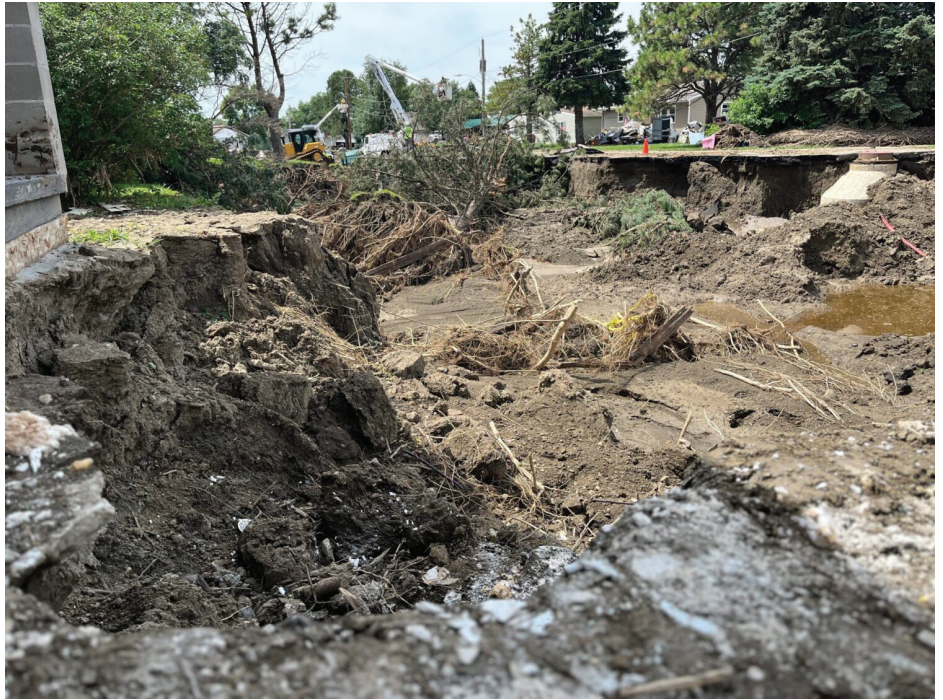
Damages remain visible in the McCook Lake community on July 3, 2024, after a massive flood hit the area on June 23. (Joshua Haiar/South Dakota Searchlight)
