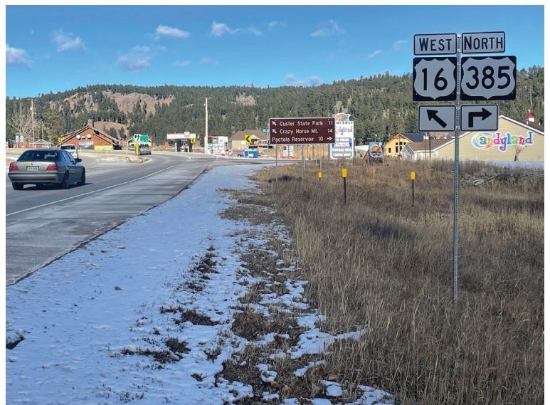
U.S. 385, shown here at its intersection with U.S. 16, is a critical link to many of the towns, attractions and businesses in the central Black Hills region. (Photo: Bart Pfankuch / South Dakota News Watch)
