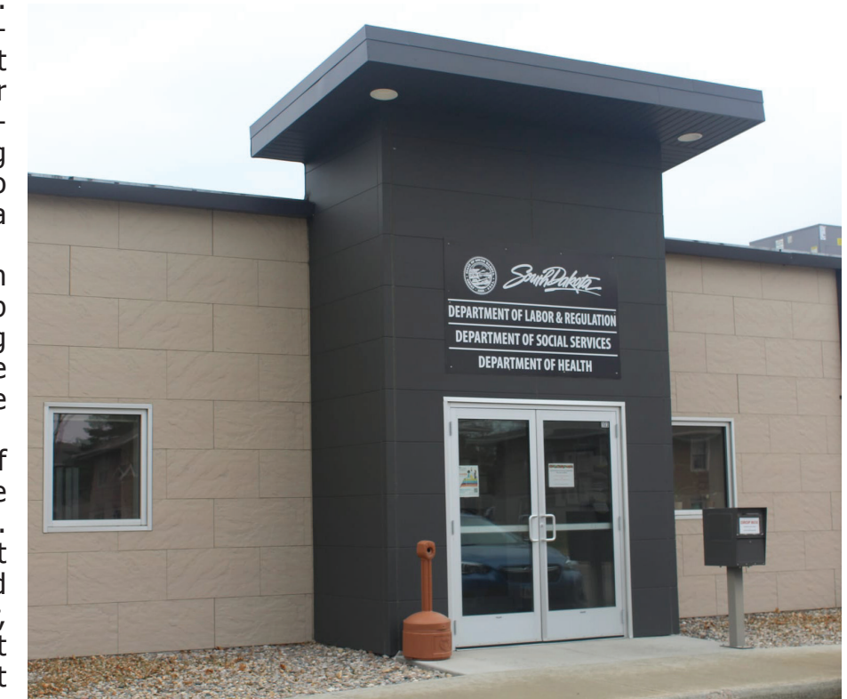
The South Dakota Department of Labor & Regulation office in Madison, S.D., is one of those that will close in February. (Photo: Jacob Boyko / South Dakota News Watch)
