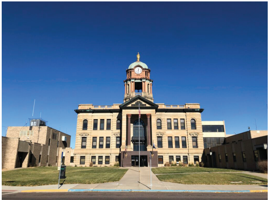
The Brown County Courthouse is located in Aberdeen and is connected to other county offices, such as the Auditor's Office and the Brown County Jail. (Makenzie Huber/South Dakota Searchlight)
