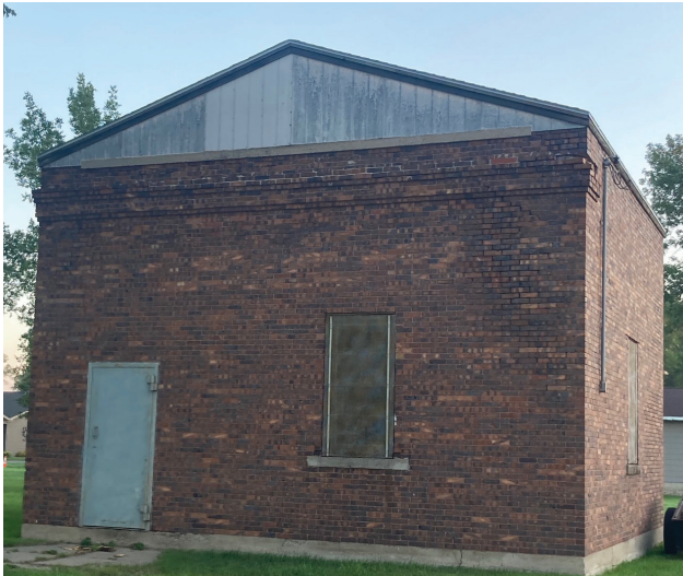
The jail building located on First Avenue in Groton. (Photo by Paul Kosel)
