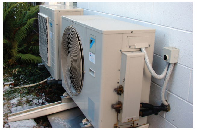
Environmentalists like heat pumps because they use a lot less energy than baseboard electric heat and oil or gas furnaces Credit: WFIU, FlickrCC.
