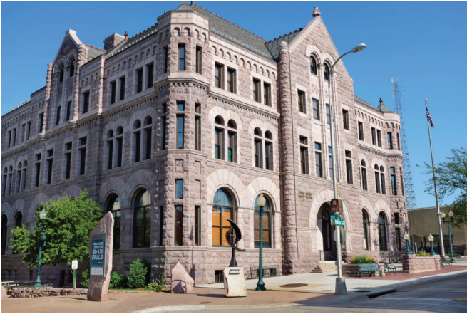
The federal courthouse in Sioux Falls, S.D.
