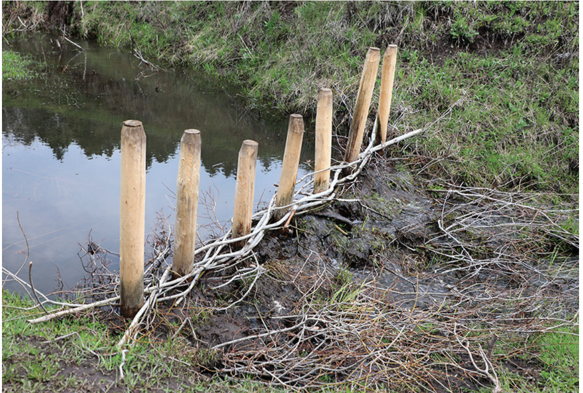
A human-made beaver dam in the Black Hills National Forest, which the Forest Service calls a "beaver dam analog." (Courtesy of U.S. Forest Service)
