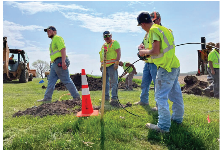
Workers lay fiber-optic cable at a broadband expansion site near Colton. (Joshua Haiar/ South Dakota Searchlight)
