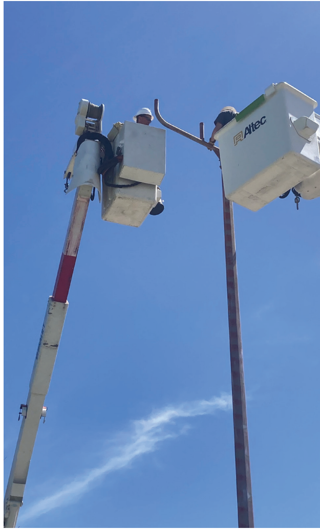
The lights at the basketball court and tennis court are operational. The left photo features Paul Kosel replacing a burnt out bulb on the tennis court. The right photo features Todd Gay and Landon Johnson having to double team to rewire the north light pole on the basketball court for the new LED fixtures.
