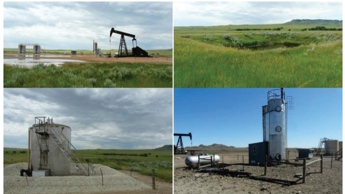
An oil derrick pump, detention pond, treatment tank and other equipment at a Citation Oil & Gas Corp. well in northwest South Dakota. (Images from SD DANR permit file)
