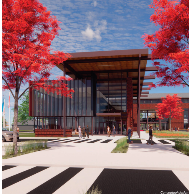
ARPA funds are being used in part to help build a new 48,000-square-foot Lincoln Hall building on the campus of Northern State University. Illustration: Northern State University
