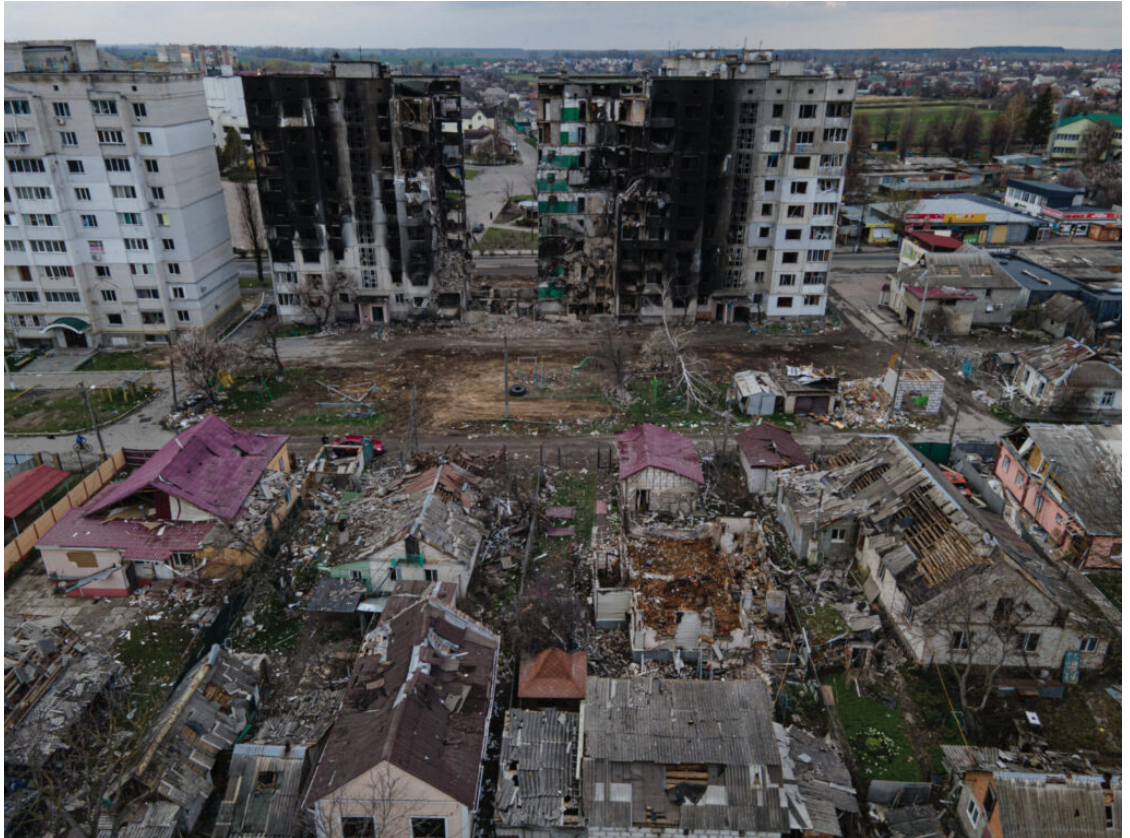
In this aerial view, a destroyed apartment building is seen next to an area of heavily damaged houses on April 21, 2022, in Borodianka, Ukraine. (Photo by Alexey Furman/Getty Images)
