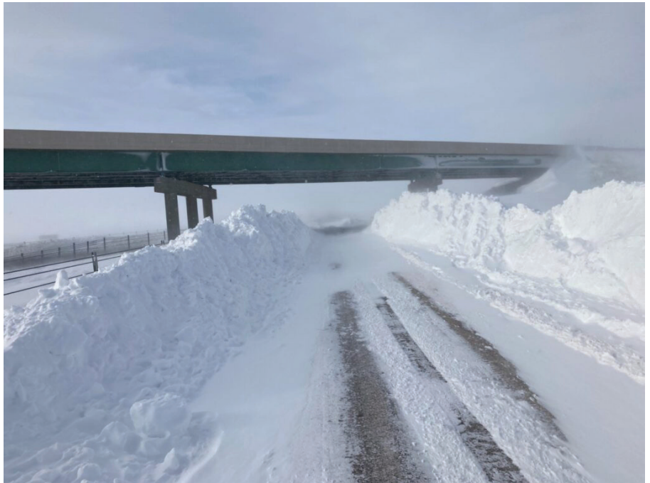
Snow piles up under an interstate bridge during a December 2022 winter storm in South Dakota. (Photo courtesy of SD
