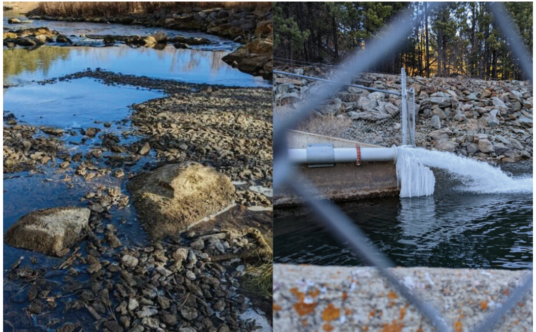
Left: The flow on Rapid Creek while a dam gate was closed at Pactola Reservoir. Right: The bypass pipe used to keep some water flowing at Pactola while the dam gate was closed. (Photos courtesy of David Hanna)
