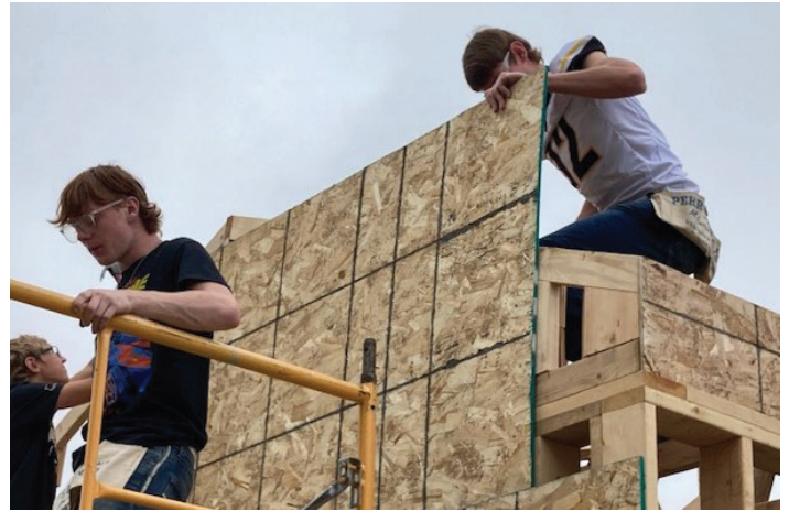
The walls are going up. (Photo by Dorene Nelson)
