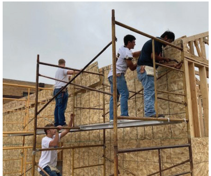
Construction continues. (Photo by Dorene Nelson)
