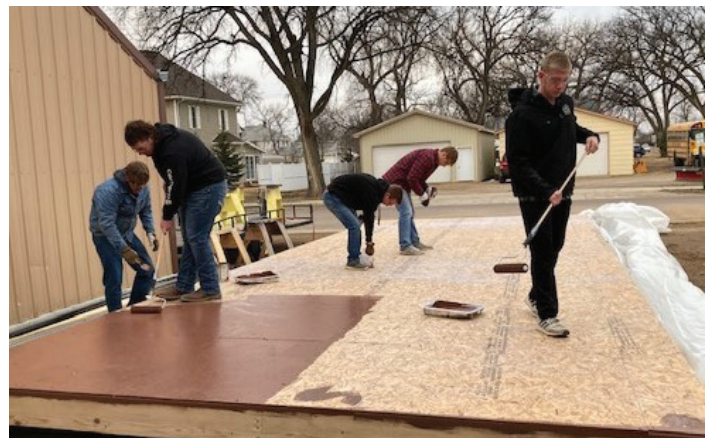
Students working on the flooring. (Photo by Dorene Nelson)
