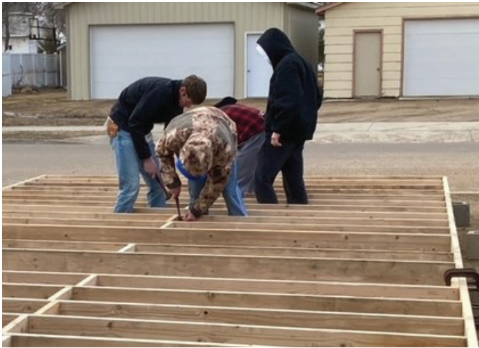
Floor joists take a lot of time. (Photo by Dorene)
