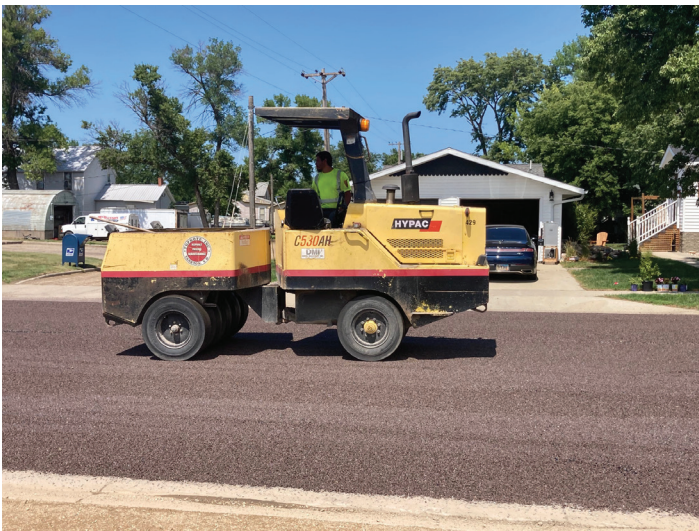
The chips are packed down.
