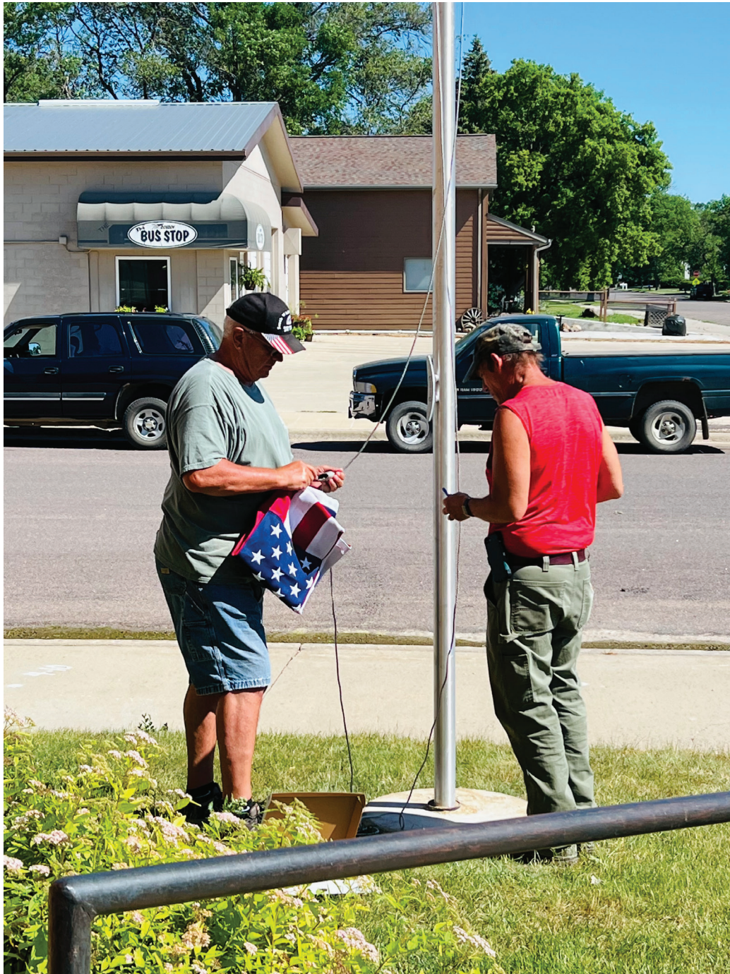
Doug Hamilton and Paul Kosel finish putting the hardware on the rope on the new flag pole at City Hall. (Photo by April Abeln)
