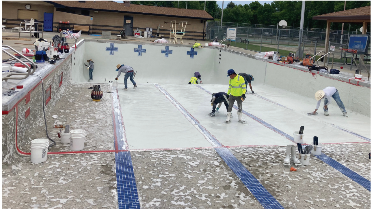
The final process of putting down the plaster was done Thursday and Friday of last week. It was then filled and the pool opened up Tuesday evening.
