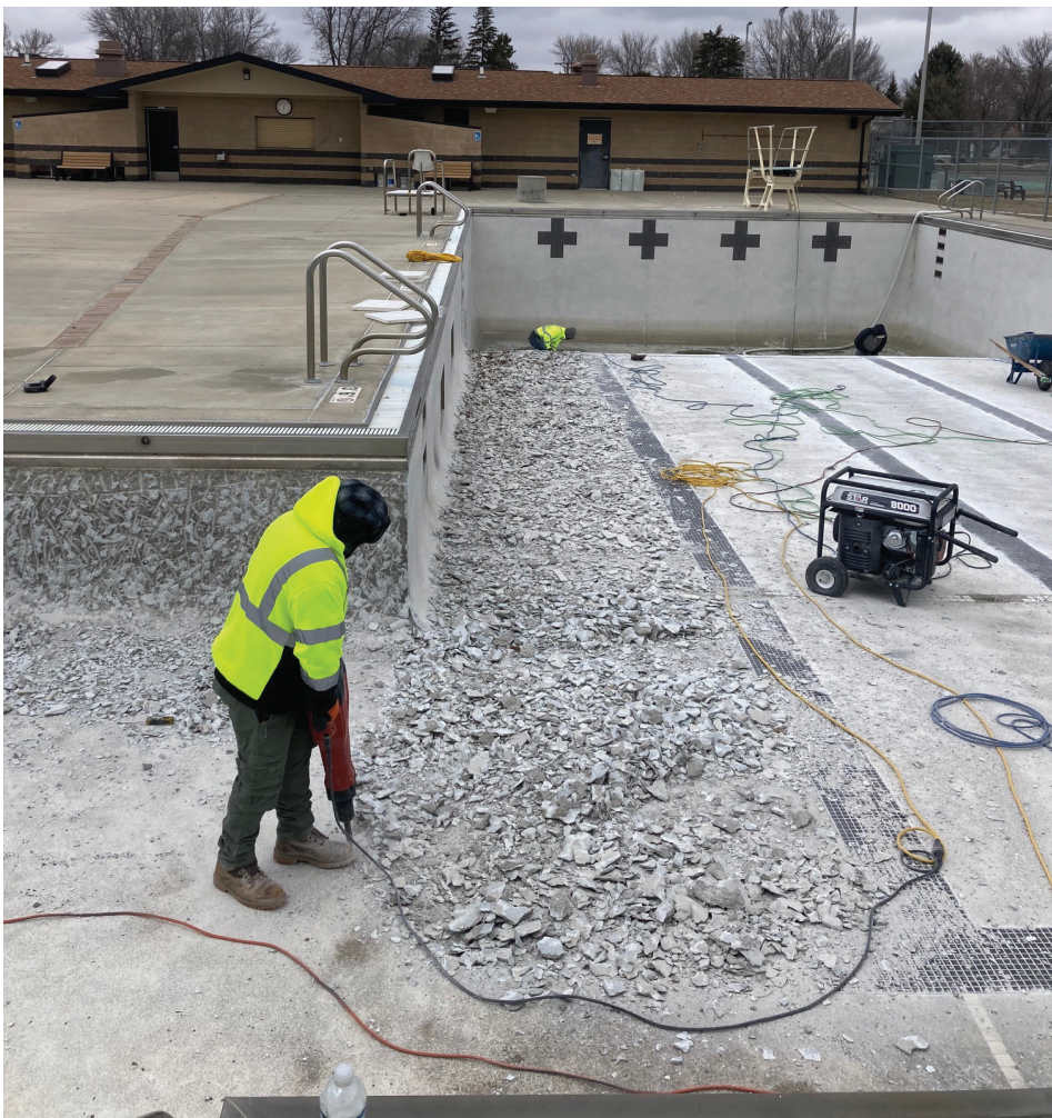
The demolition of the Groton pool has begun. The plaster will be removed and replaced later this month. (Photo by Paul Kosel)
