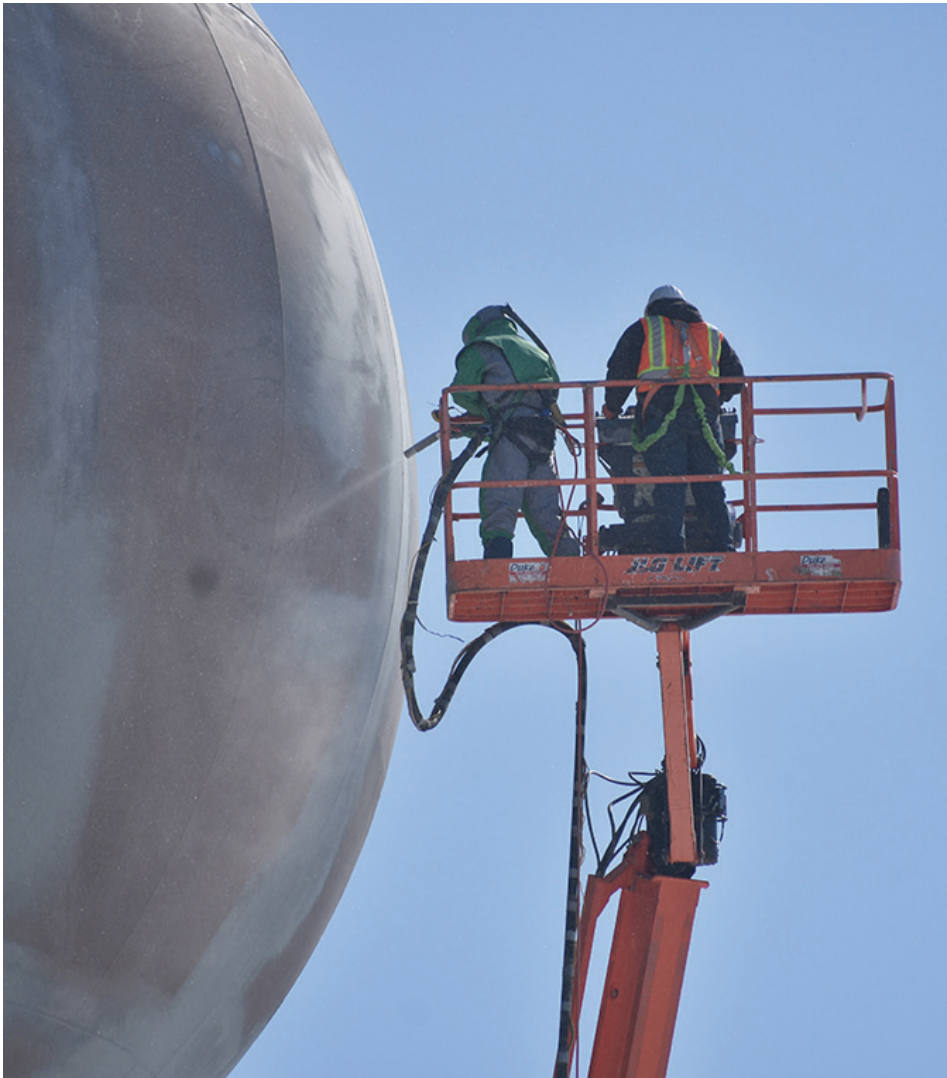
Sandblasting of the new water tower continued last week as the tower is being prepped for painting. If all goes well, priming of the tower was also started on the inside. The actual painting will have to wait until air temperatures are at least 40 degrees, day and night. (Photos by Paul Kosel)
