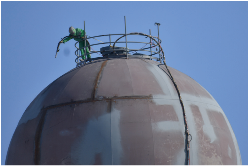
Sandblasting of the new water tower continued last week as the tower is being prepped for painting. If all goes well, priming of the tower was also started on the inside. The actual painting will have to wait until air temperatures are at least 40 degrees, day and night. (Photos by Paul Kosel)
