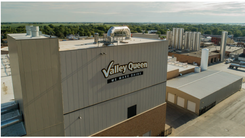
The Valley Queen Cheese factory in Milbank, South Dakota recently underwent a $52 million expansion that created the need for millions more pounds of milk from dairy farmers in South Dakota. Photo: Courtesy Valley Queen Cheese
