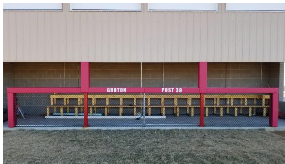
Finishing touches just went up on the Locke-Karst Field dugouts! Check out the new rail pads. (Photo from Groton Baseball/Softball Foundation Facebook Page)
