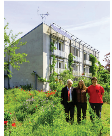
Dr. Wolfgang Feist and family pose in front of the world's first passive solar house, constructed in 1991 in Darmstadt, Germany.
