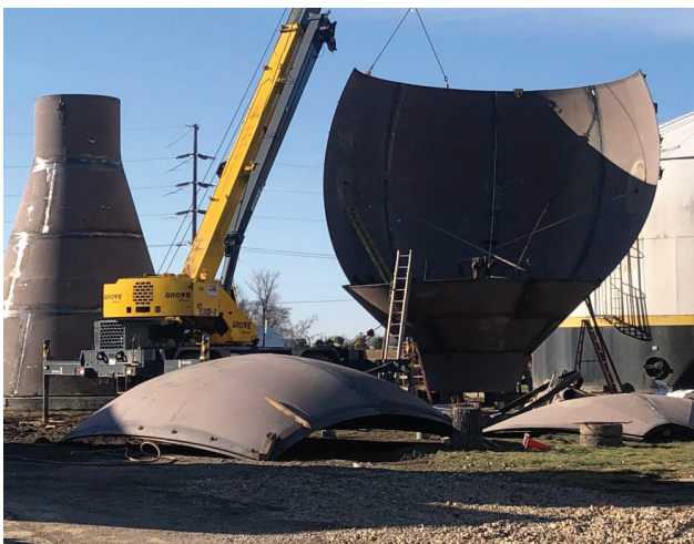
The bowl to the water tower was assembled on Wednesday. As work continues to progress, the crew is working seven days a week and as soon as the bowl is fully assembled, the big crane will arrive in Groton as the sections to the tower will then be assembled. (Photo by Paul Kosel)
