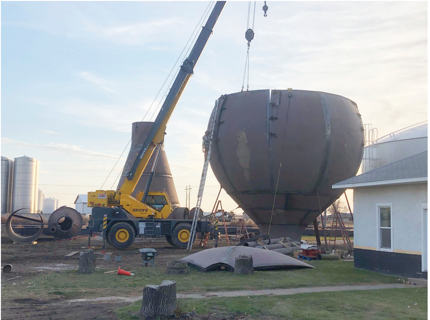
The bowl to the water tower was assembled on Wednesday. As work continues to progress, the crew is working seven days a week and as soon as the bowl is fully assembled, the big crane will arrive in Groton as the sections to the tower will then be assembled. (Photo by Paul Kosel)
