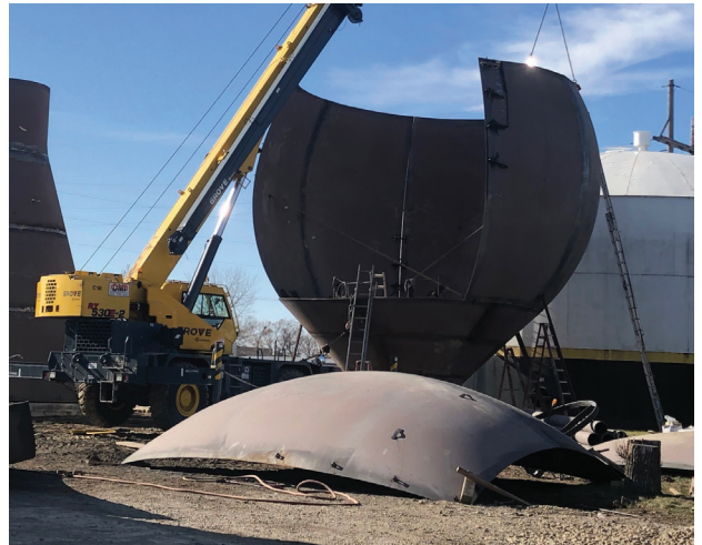
The bowl to the water tower was assembled on Wednesday. As work continues to progress, the crew is working seven days a week and as soon as the bowl is fully assembled, the big crane will arrive in Groton as the sections to the tower will then be assembled. (Photo by Paul Kosel)
