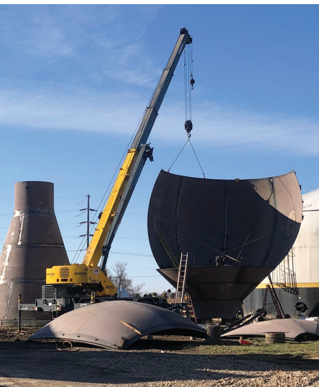
The bowl to the water tower was assembled on Wednesday. As work continues to progress, the crew is working seven days a week and as soon as the bowl is fully assembled, the big crane will arrive in Groton as the sections to the tower will then be assembled. (Photo by Paul Kosel)
