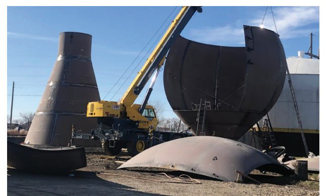
The bowl to the water tower was assembled on Wednesday. As work continues to progress, the crew is working seven days a week and as soon as the bowl is fully assembled, the big crane will arrive in Groton as the sections to the tower will then be assembled. (Photo by Paul Kosel)
