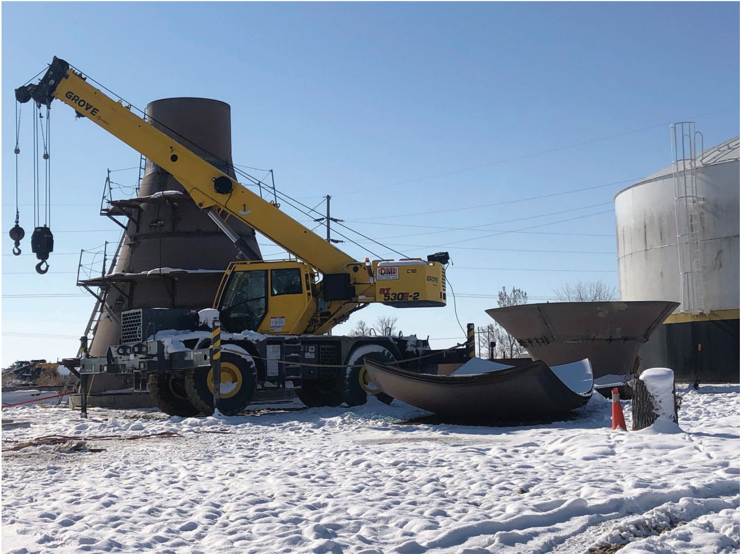
Another section of the water tower was assembled on the ground.
