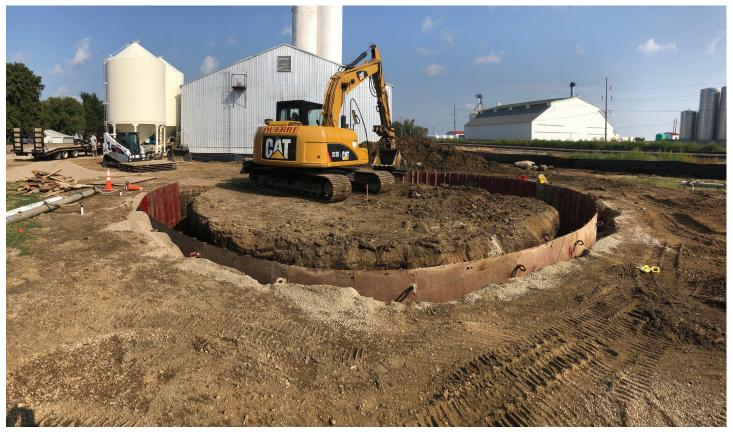
The hole is being dug for the footing for the new water tower.
