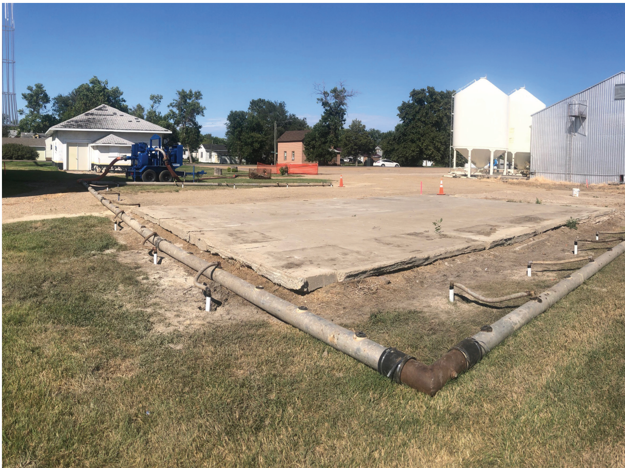
Dewatering has begun for the new water tower A big pump has been operating 24 hours a day at the site of the new water tower. You can see the big pipes above the ground with several white pipes in the ground as the area is dewatered for the new footings of the water tower. The new water tower will be about the same height as the existing one at 140 feet. The current tower holds 80,000 gallons while the new one will hold 125,000. (Photo by Paul Kosel)
