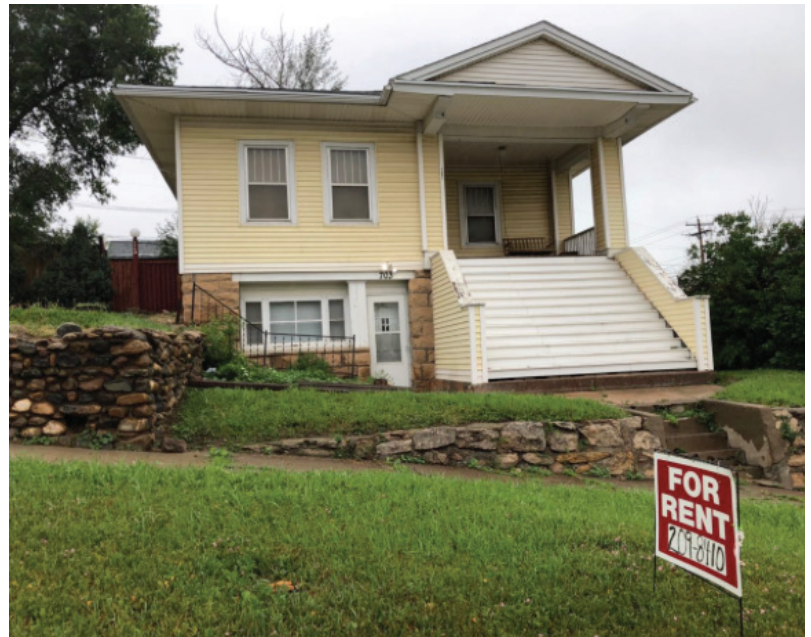
Prior to the pandemic, a third of South Dakotans were considered "rent burdened," meaning they were paying 35% or more of their monthly income on rent and therefore unable in many cases to afford a nice rental home, such as this one in Rapid City. Photo: Bart Pfankuch, South Dakota News Watch
