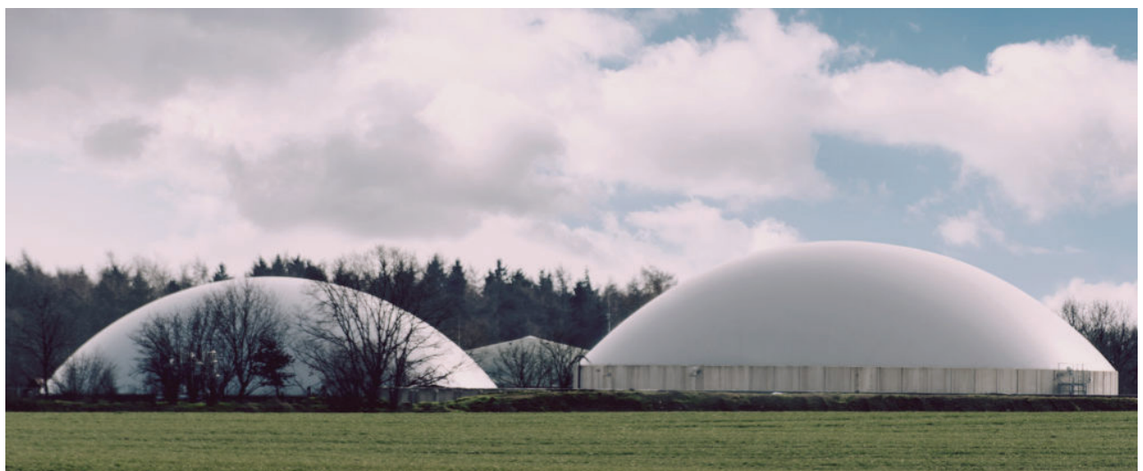
Anaerobic digesters, such as those pictured here, provide an ideal environment for microorganisms called methanogens to digest manure and produce methane that can be harvested, filtered and sold as natural gas. Three Sioux Falls-area dairy farms will become home to similar digesters within the next two years. Photo: Submitted
