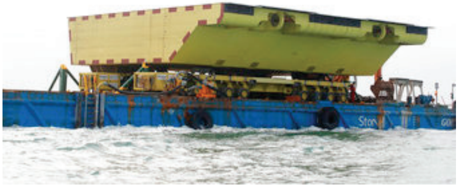
A yellow barrier, part of a plan to protect the city of Venice from flooding, floats on a barge, in Venice, Italy, Friday, Nov. 29, 2019. Central to the plan to protect Venice, some, or all, of the 78 barriers will one day be raised when the sea rises more than 110 centimeters to prevent damaging high tides from pushing into the lagoon city, a UNESCO heritage site built picturesquely but somewhat precariously among more than 120 islands. (AP Photo/Antonio Calanni)
