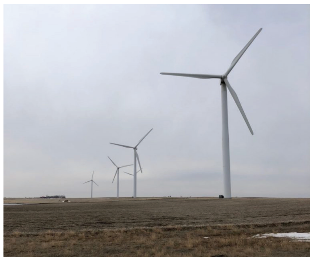
These wind towers are part of the state's first wind farm built south of Highmore in Hyde County in 2003. These older towers are 213 feet tall, while modern towers now being built are often more than double that height. Photo: Bart Pfankuch, South Dakota News Watch
