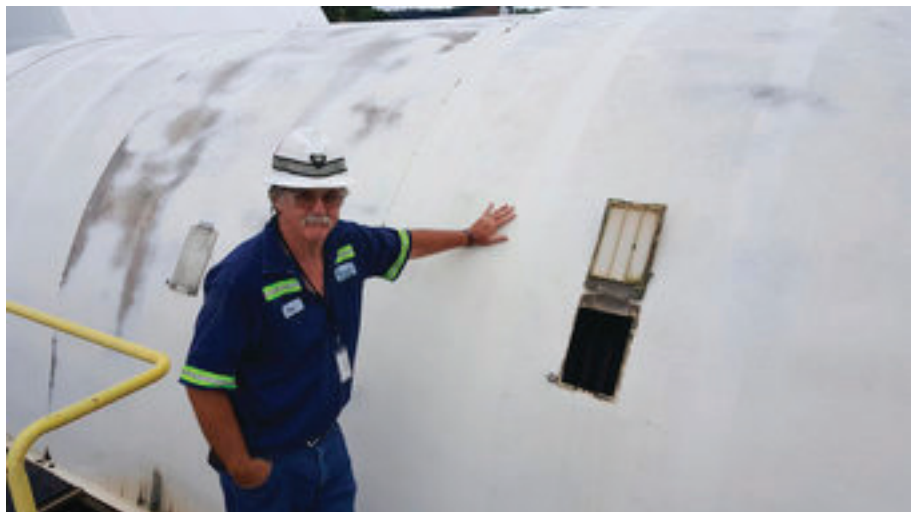
Ken Noren, foreman at the wastewater treatment plant at Sanford Lab, stands next to one of the filtration systems, which uses bacteria to remove ammonia and other pollutants from water siphoned from underground on Aug. 5, 2019 in Lead, S.D. Ever since the wastewater treatment plant reopened in 2008, the Sanford Underground Research Facility located on the Yates Shaft campus has been making improvements and modifications to its treatment process. (Alex Portal /Black Hills Pioneer via AP)
