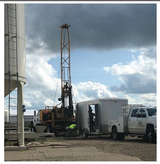
Drilling for soil samples at the proposed site of the new water tower has begun. The city will be putting up a new one next year. Soil samples are being taken east of the reservoir. (Photo by Paul Kosel)
