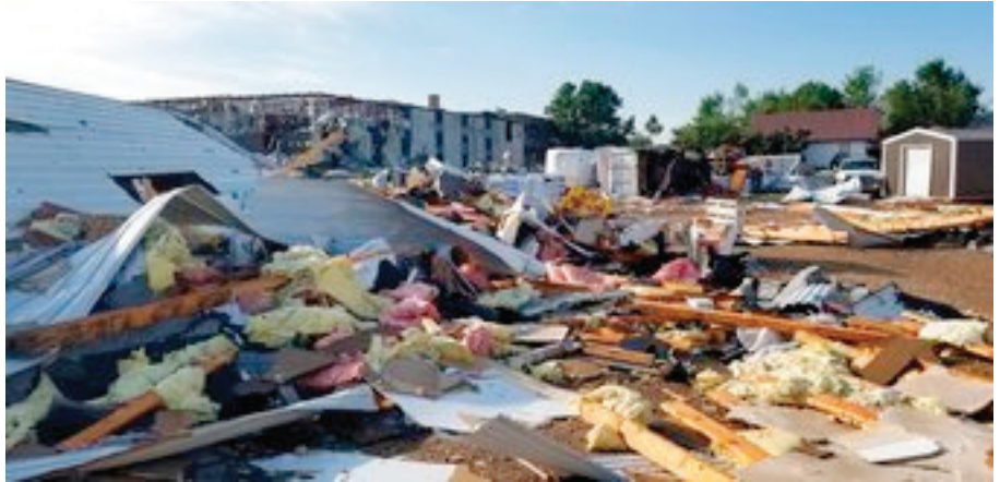
A lumberyard was destroyed in Burke, South Dakota after a severe thunderstorm blew through the area on Tuesday, Aug. 6, 2019. (Jason Witt/The Argus Leader via AP)
