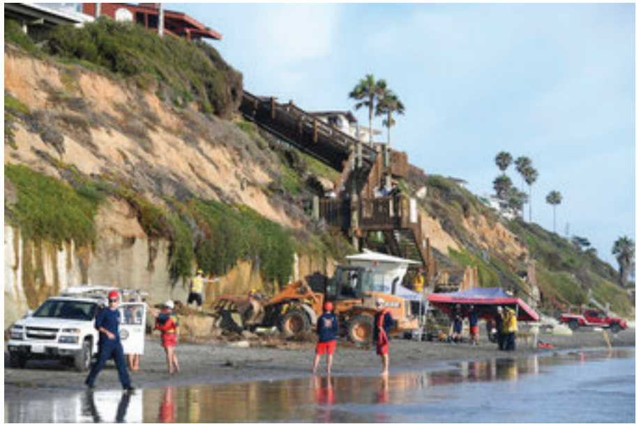
Search and rescue personnel work at the site of a cliff collapse at a popular beach Friday, Aug. 2, 2019, in Encinitas, Calif. At least one person was reportedly killed, and multiple people were injured, when an oceanfront bluff collapsed Friday at Grandview Beach in the Leucadia area of Encinitas, authorities said. (AP Photo/Denis Poroy)
