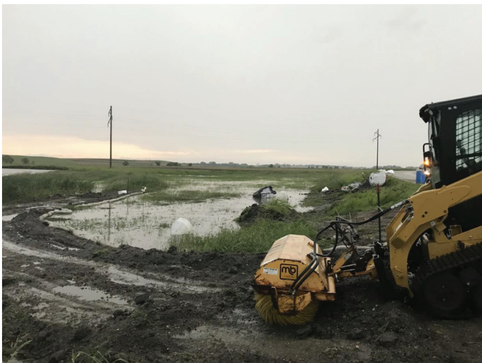
The day after the June 26 crash, a bulldozer built an earthen berm around the area in an unsuccessful attempt to prevent spilled chemicals from entering the Big Sioux River, visible at upper left. Photo: Courtesy EPA
