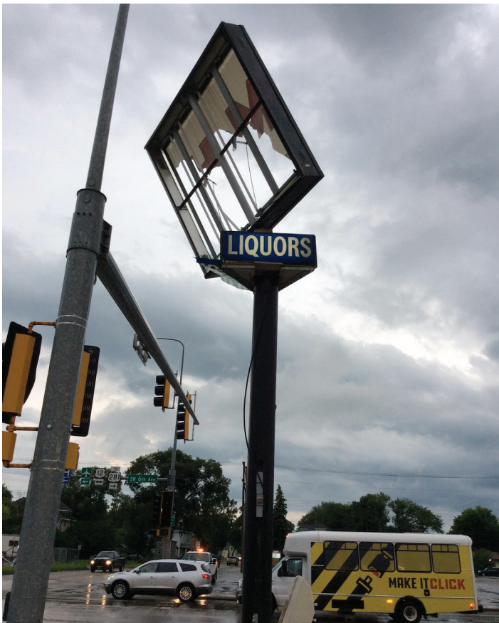
Business Marquee Sign Damage in Aberdeen, SD. Photo Credit: NWS Aberdeen.
