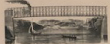
Railroad Bridge, Reading Railroad, New York, 1845
