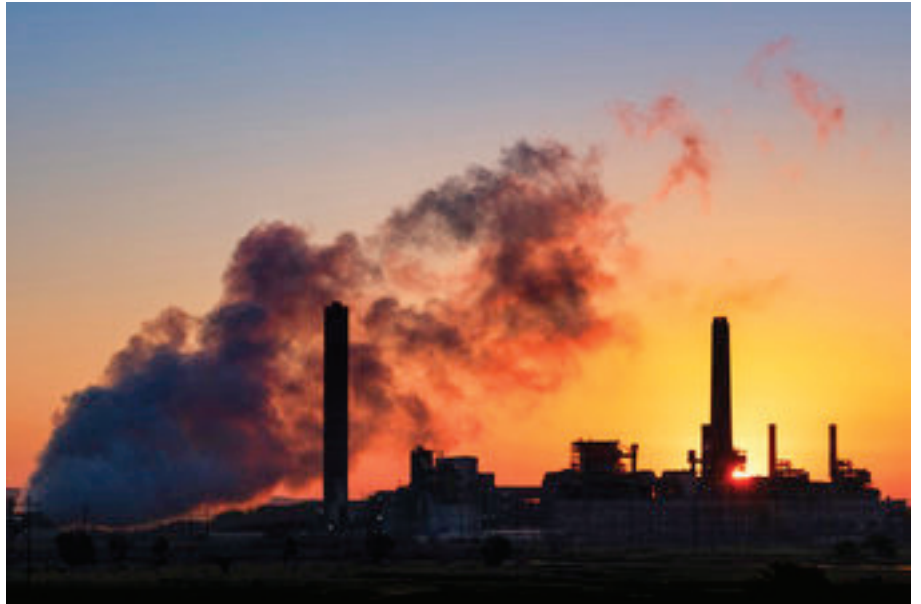
FILE - In this July 27, 2018, file photo, the Dave Johnson coal-fired power plant is silhouetted against the morning sun in Glenrock, Wyo. The Trump administration is close to completing one of the biggest of its dozens of rollbacks of environmental rules, replacing a landmark effort to wean the nation's electrical grid off coal-fired power plants and their climate-changing smokestack emissions. (AP Photo/J. David Ake)
