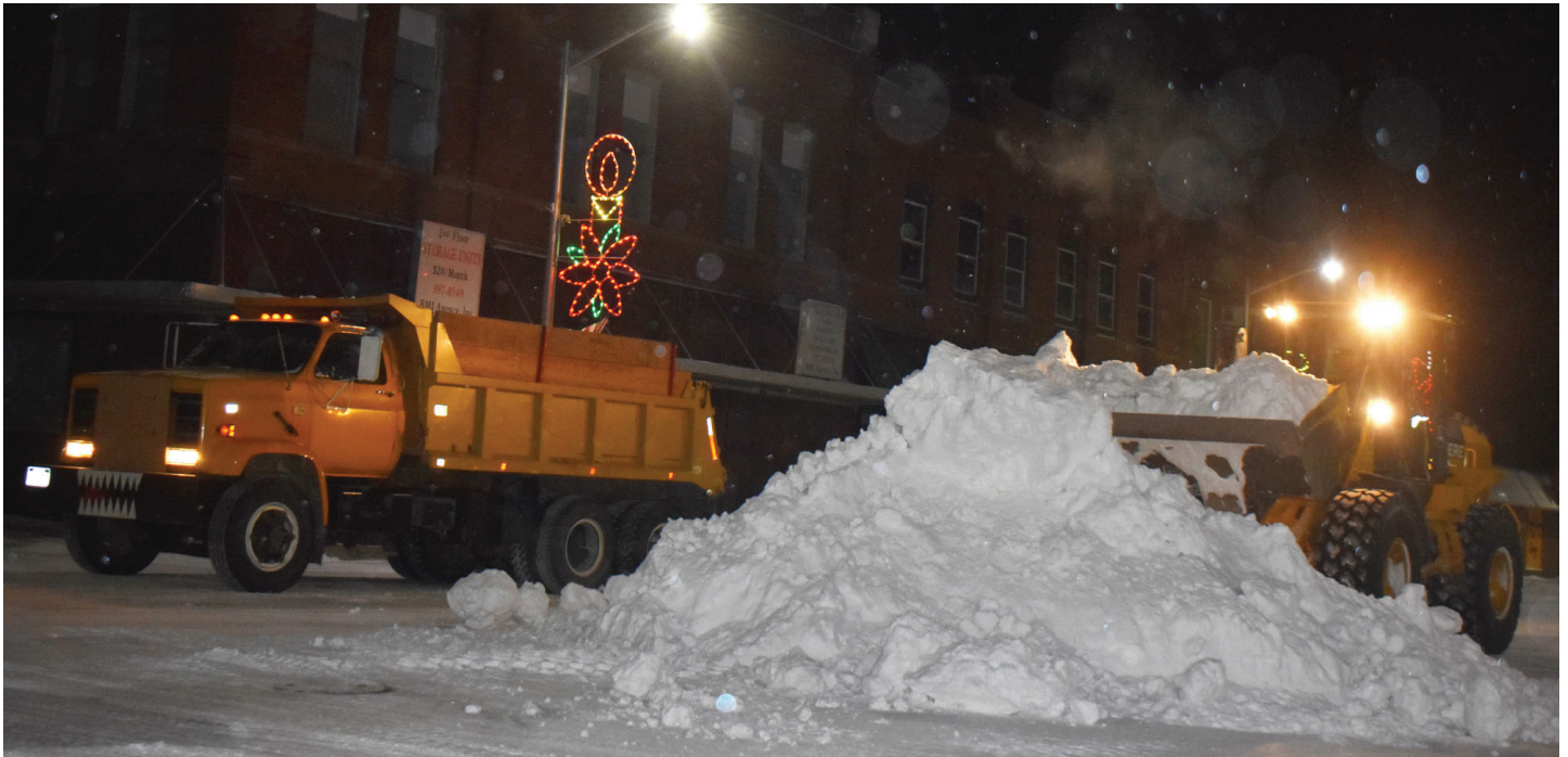
The city crew was out this morning hauling off many truck loads of snow off of Groton's Main Street. (Photo by Paul Kosel)
