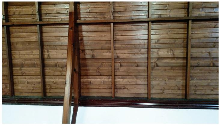
By mid-morning Wednesday, the crew re-roofing Historic Trinity Church had installed the new rafters and ceiling boards, covering the huge hole where rotted ceiling boards and two rafters were removed the day before.
