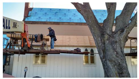
After installing the new ceiling boards and rafters, the crew covered them with a layer of half-inch plywood to provide a sturdy base for the new steel shingles. The blue layer on the top of everything is a moisture barrier underlayment.
