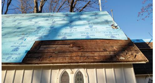
The three layers of old shingles on the South roof, including the original 1884 wooden ones, were removed except for the lower SE corner, which had rotted out so much that light coming through the roof is visible from the inside. The roofing and ceiling boards will be torn off and replaced like the North roof ones were, except in a much smaller area. (Photo
