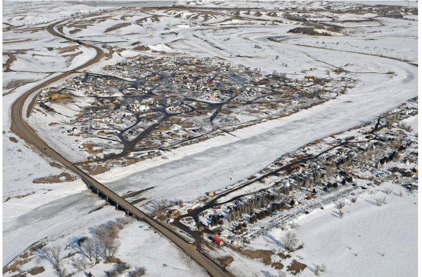
This aerial photograph shows North Dakota highway 1806 at left where it crosses Cannonball River and protest camps on both sides of the river during the Dakota Access Pipeline protest in February 2017. Some South Dakota officials are concerned over a state law that requires counties to pay a significant amount for protest activities before the state steps in with financial help. It cost more than $40 million to handle the protest in North Dakota. (Photo by Tom Stromme, courtesy of Bismarck Tribune)
