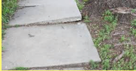
NEW OR REPLACED SIDEWALK
