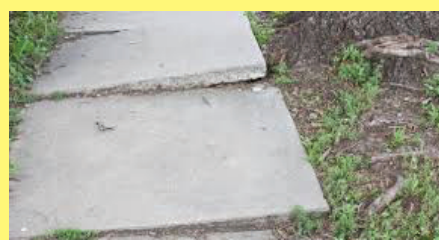
NEW OR REPLACED SIDEWALK
