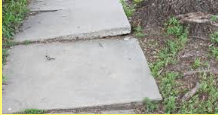
NEW OR REPLACED SIDEWALK
