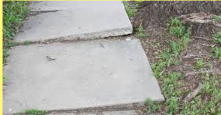
NEW OR REPLACED SIDEWALK
