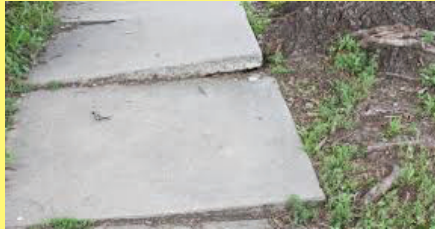
NEW OR REPLACED SIDEWALK
